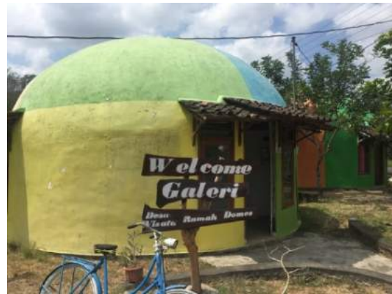
Dome house built as part of disaster reconstruction
